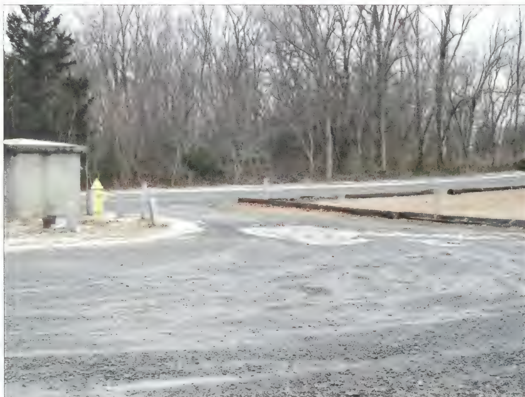
Figure 3.24. View looking west at entry to parking area, Battery Potter. Southwest of the main entry, a small parking area departs from Hudson Drive, loops around a small building, and joins back up with Hudson Drive (Olmsted Center, January 2009).
